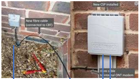
New external incoming junction box installed externally and normally towards "Front of Property"
